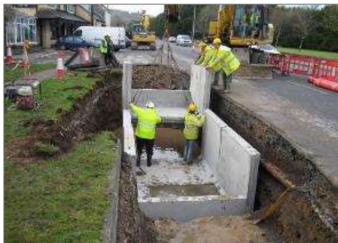
Figure 8 - Standard joint bay under construction (pre-cast)
