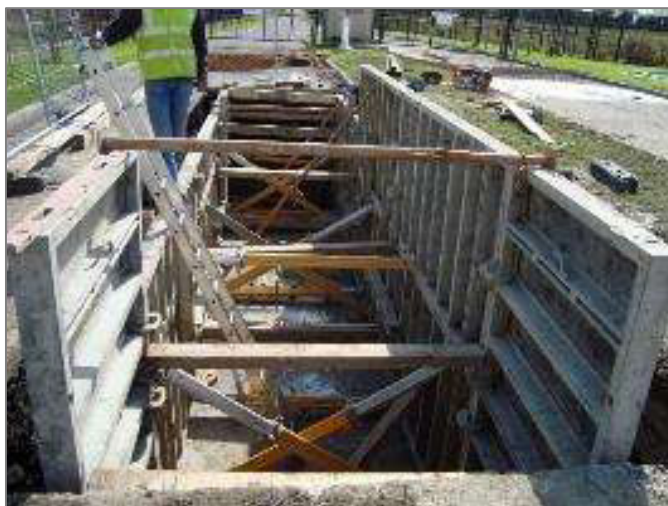
Figure 6- Standard joint bay under construction (in-situ)
