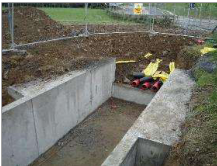
Figure 7 – Example of completed joint bay prior to cable installation (in-situ)
