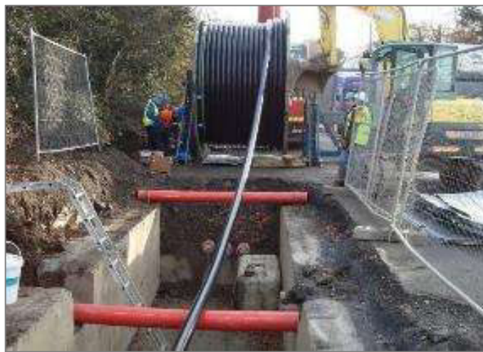
Figure 9 - HV cable pulling procedure (Standard drum set-up)
