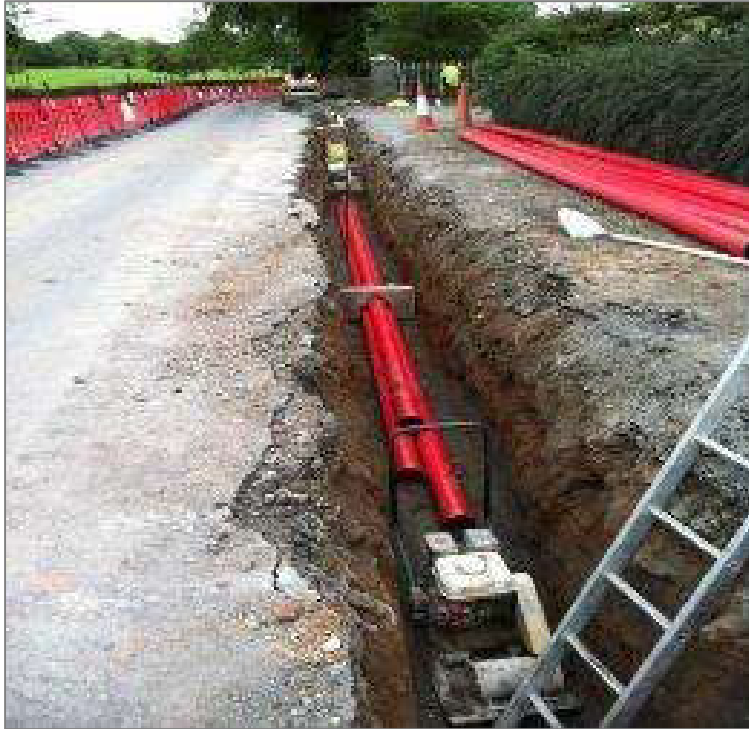
Figure 2 - Standard 110kV Underground Duct Installation
