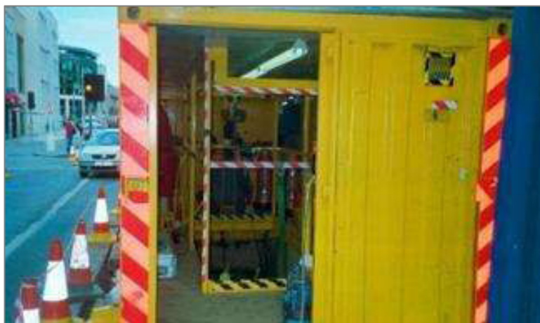
Figure 10 - HV cable jointing container
